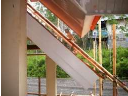
Barge boards on roof line repainting/woodwork that has been stripped back ready for recoating
