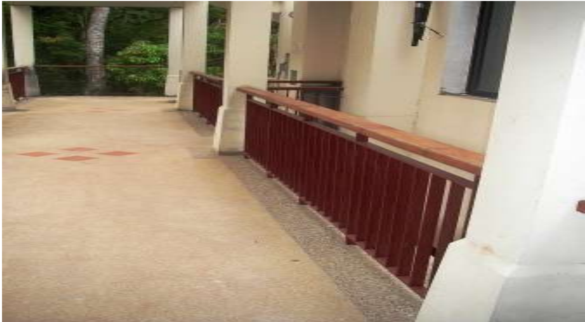
Anti rust and sanding of railings/handrail ongoing on walkways/balconies
