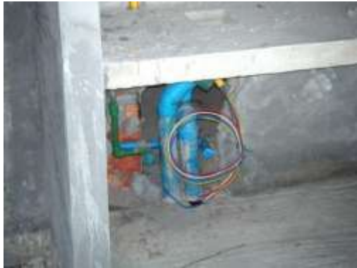
The plumbing rework completed in bathrooms (raise water heater fittings)/view across from 8A
