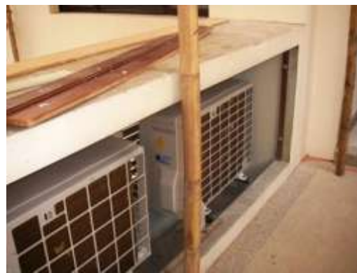
Working on modification to Sala/ New compressors fitted to standard units (bedroom units)
