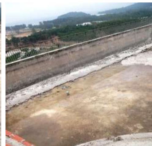
Preparation works to the roof top pool to prepare for tile installation
