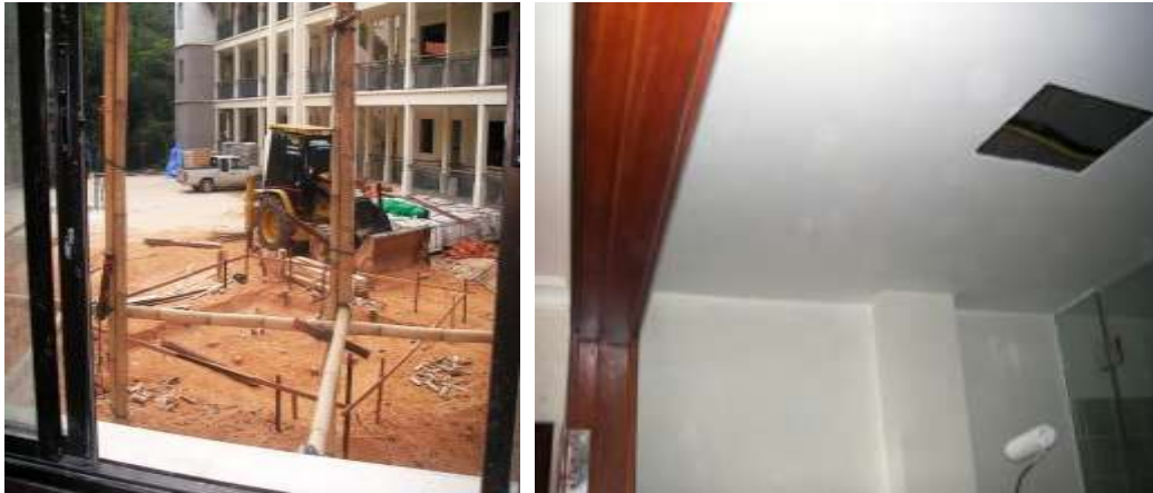
View outside from Lg 1 toward Lemongrass 2/ ceiling being repainted Lg1 9B
