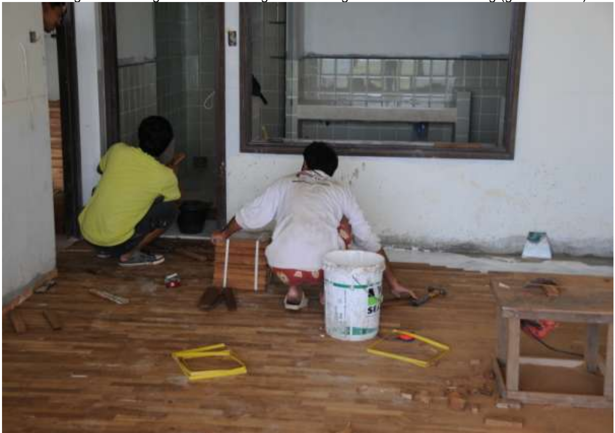
Laying parquet flooring in Lemongrass 2
