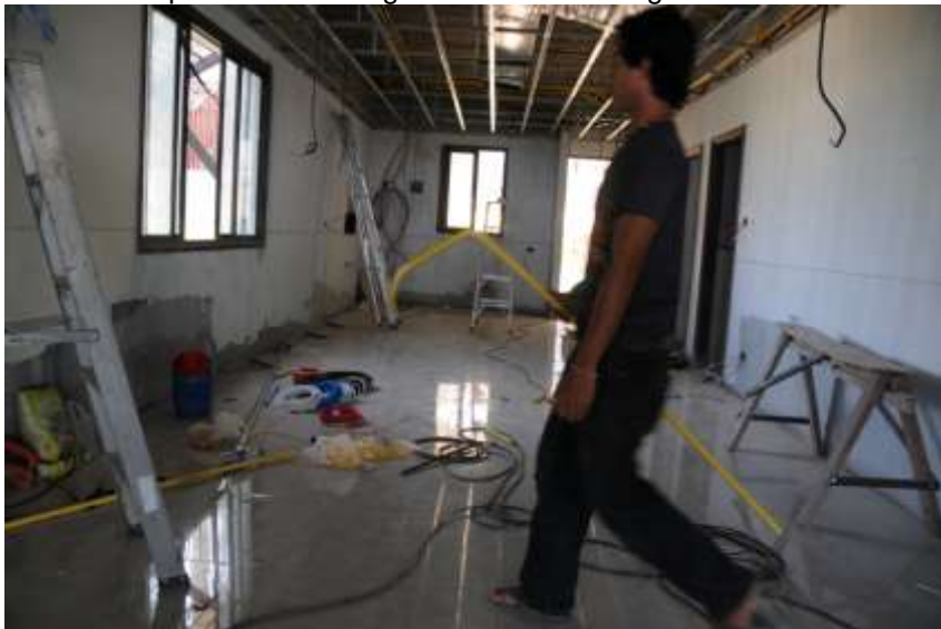
Air con engineers at work in Lg 2 with the Electricians Regards,
