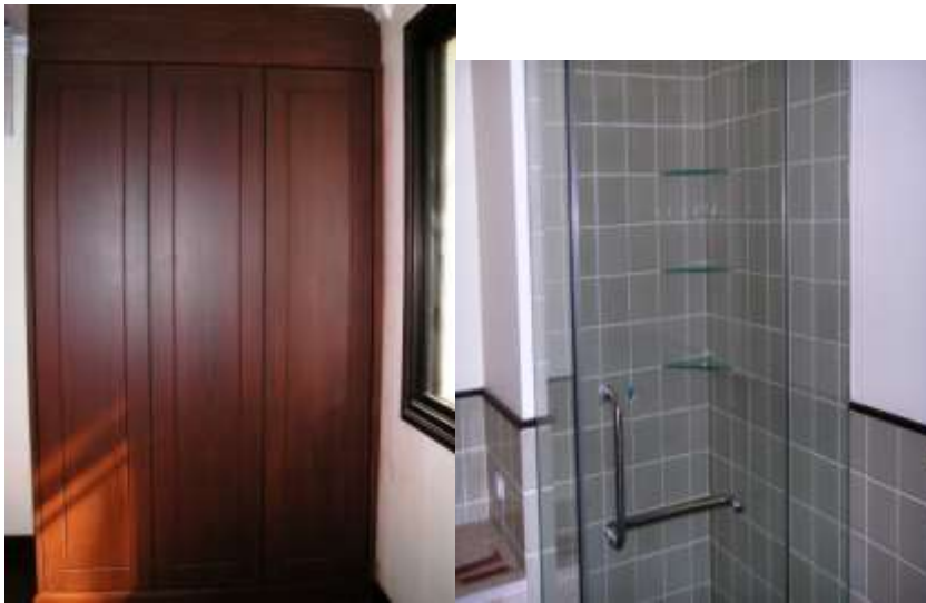
Wardrobes in lemongrass 1 nearing completion, glass shelving fitted to shower cubicles
