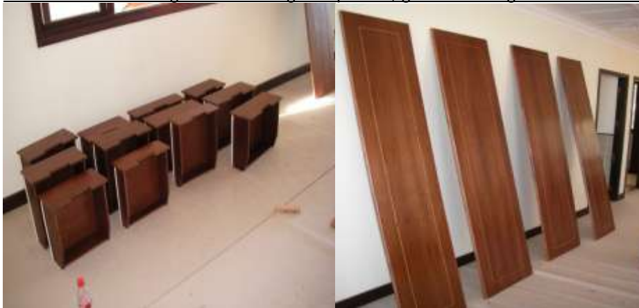
Work in progress on drawers and doors for wardrobes in Lemongrass1
