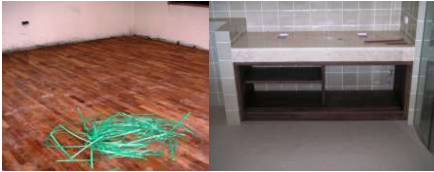
Parquet flooring being installed & Installation of under sink cabinets in bathrooms
