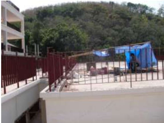
Railings on roof terrace completed awaiting hand rail installation/ ongoing interior decoration
