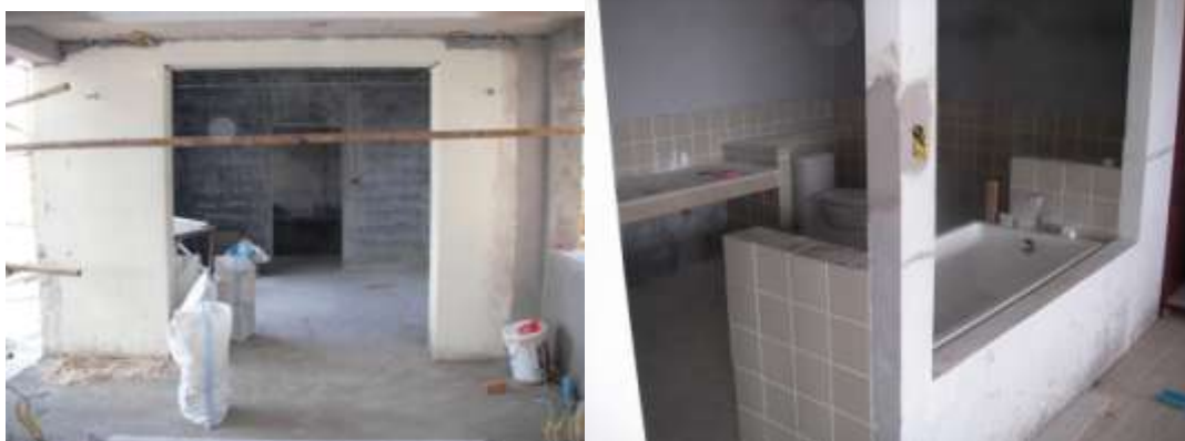
Lg2 6B Master bedroom entrance(modified)/6b bath installed in 2 nd Bedroom
