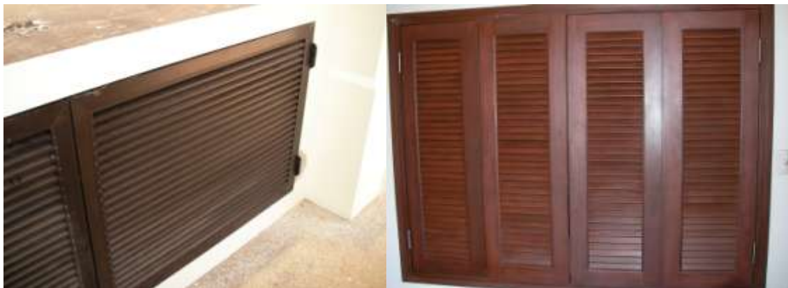
Air con compressor vent covers/shutter dividing master bath/master bedroom
