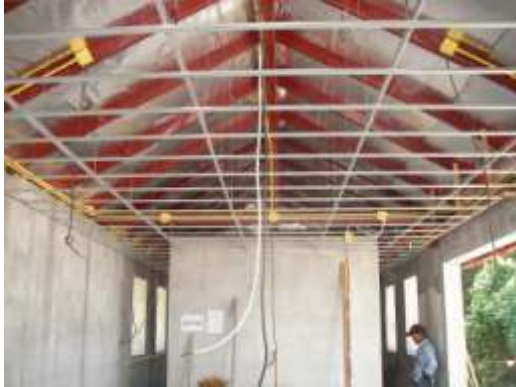
Installing framework for ceiling 12C and the roof tile colour change master bedroom 12C
