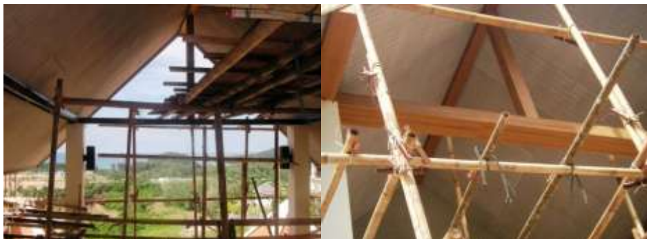
Left picture shows steelwork exposed, right picture shows the new wooden surround to hide steel
