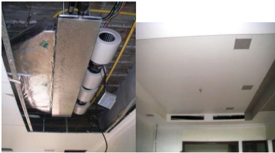
Air handling unit (living)/ceiling work for Air con system
