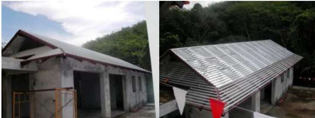
Steel roofing works to 12c now completed.
