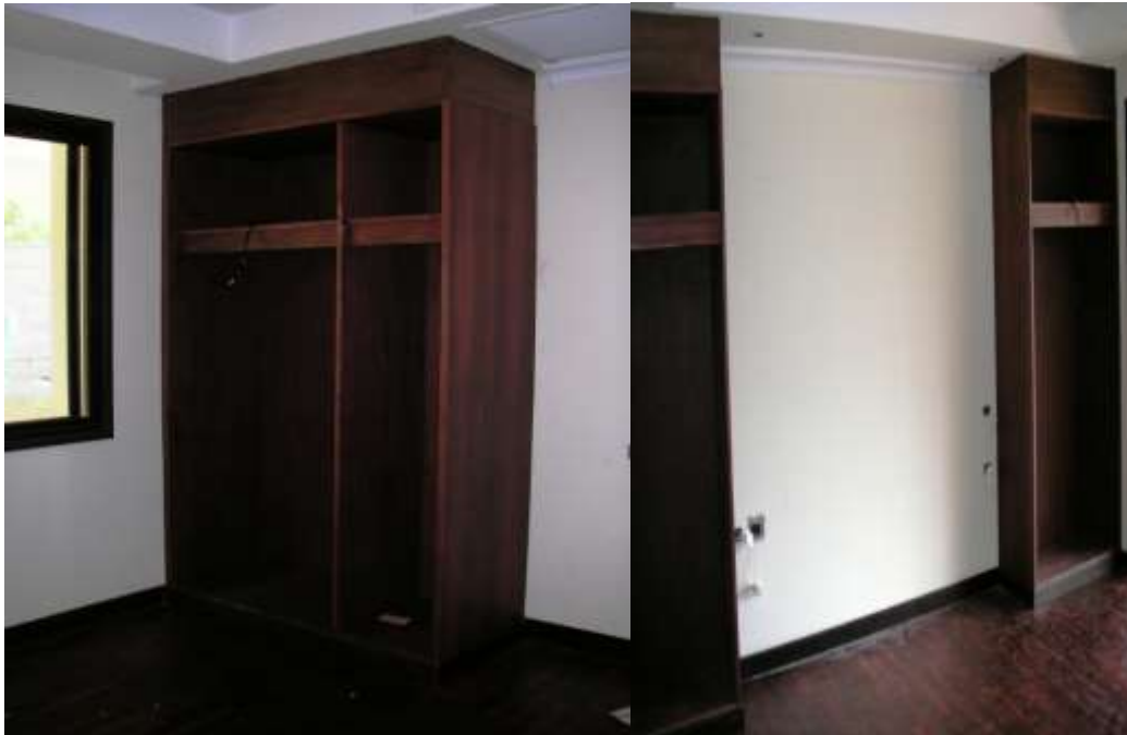
Wardrobes in Lemongrass 1 in various stages of completion.
