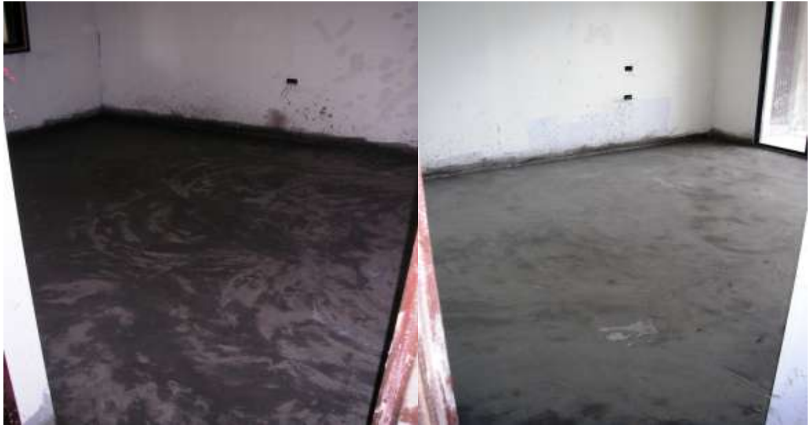
Cement flooring relaid after chipping(above) ready for parquet flooring installation.
