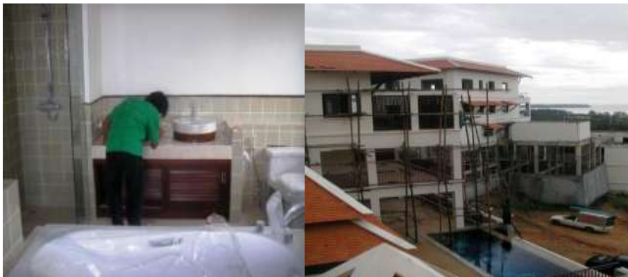
Worker finishing the wood on basin surround/erecting scaffold Lemongrass 1
