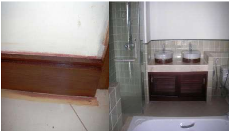
New lighter woodwork finish/Decorative surrounds for wash basin
