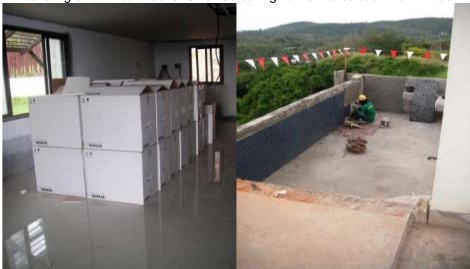
Sanitary systems arriving on site for fitting/Lg2 33B pool tile installation
