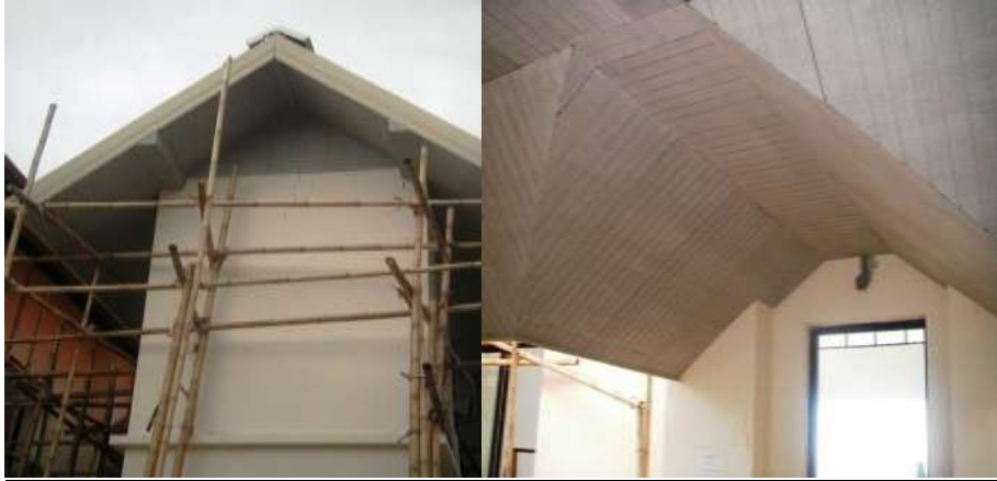
Roofing works on upper walkway and entrance to Penthouse units
