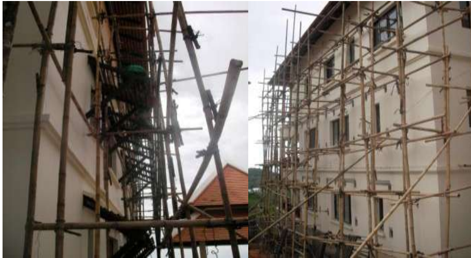
Side Steel work modification works in Lemongrass 1
