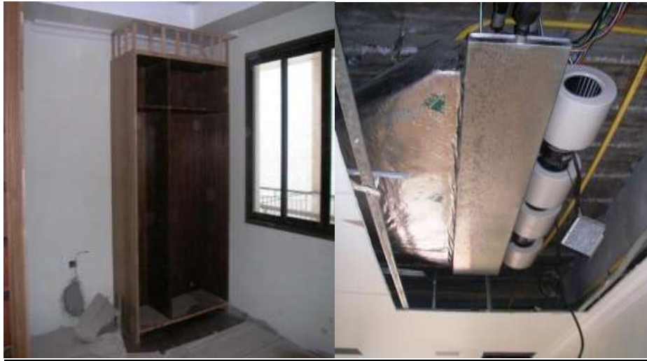
Wardrobes in various finishing stages/Air handling unit (living)
