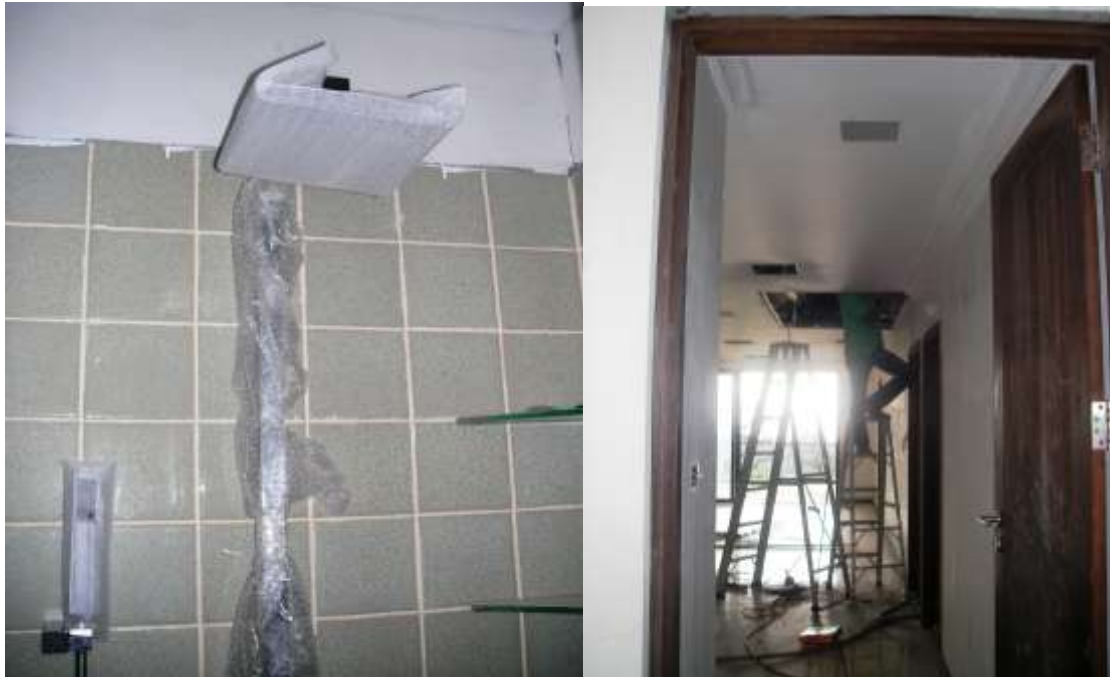
Sanitary fittings being installed/ work ongoing on Air con systems
