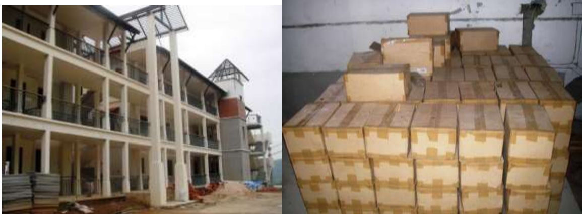
View of back of Lemongrass 2 blocks A and B/Pool tile for the pools with units on this block
