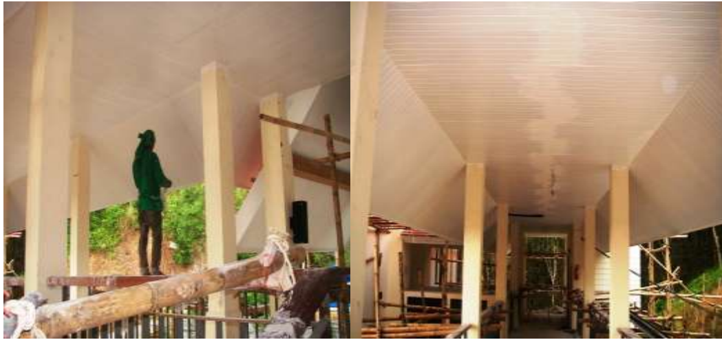
Painting of the walkways ceiling is ongoing
