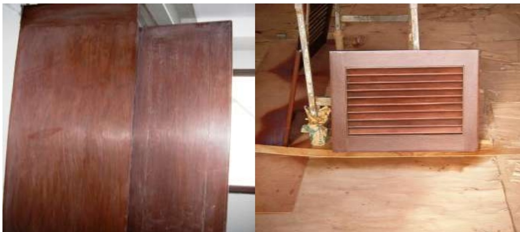
Finishing of wardrobes and doors for under sink counter units
