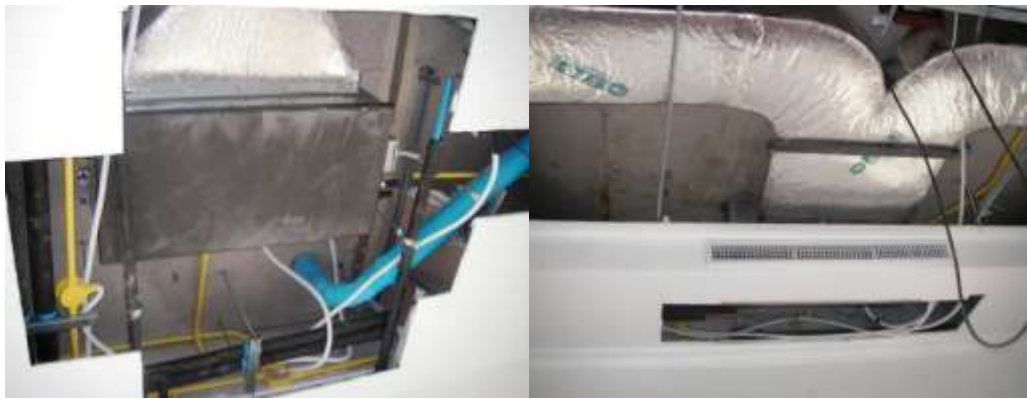
Work on Penthouse Air con system modification
