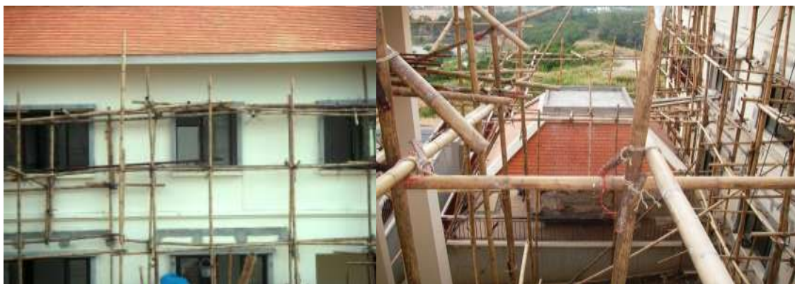
Barge boards painted/lintle around windows installed/modified salas roof line
