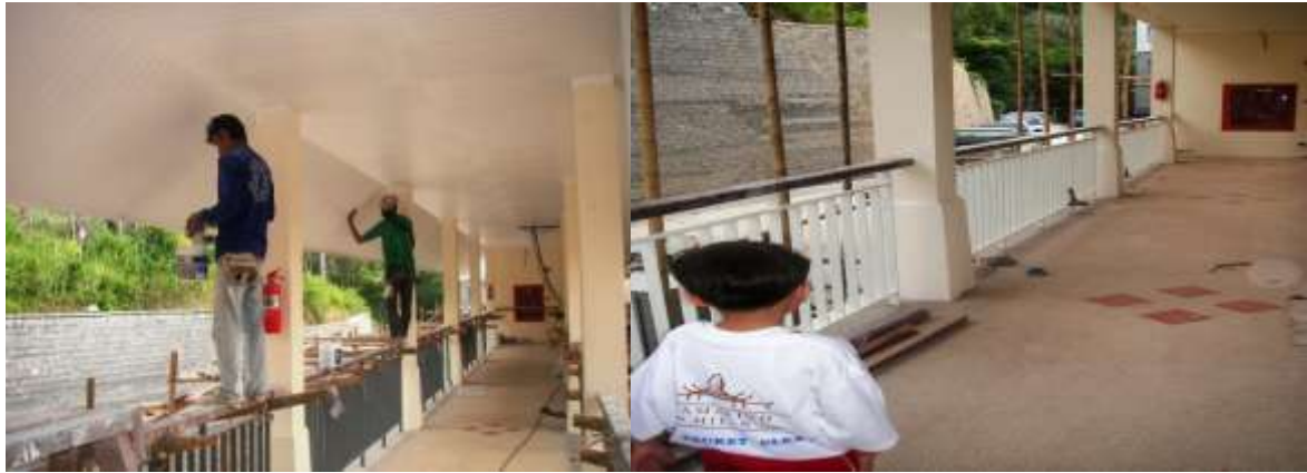
Walkway ceilings being painted/undercoat applied to railings on walkway
